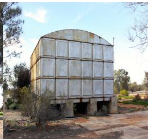
Rainwater storage tank. Rainwater is collected from the aircraft parking bay at the Maralinga airstrip, directed into a storage dam for settling, then pumped into storage tanks. These tanks are original, they are made of panels bolted together, and they are huge !
